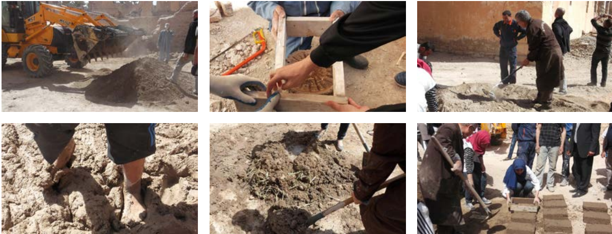
Figures 3a-f. The stages of adobe production during the restoration of the ksar of Lichana in 2015 (photos S. Zerari, V. Pace, L. Sriti, 2015).
