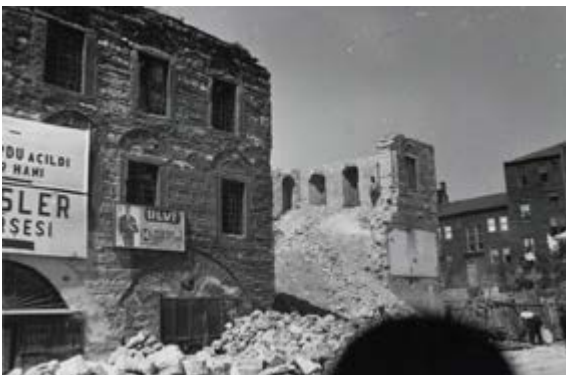
Figure 20. Istanbul. Destruction of Simkeşane. Salt Research Archive, Archive No. TASUH7029003 ( https://archives.saltresearch.org/handle/123456789/76798 , access June 15 th 2019).
