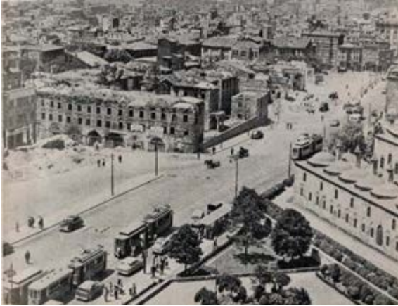
Figure 18. Istanbul. Simkeşane and Ordu Avenue before the demolition (UNSAL 1968, p. 33).
