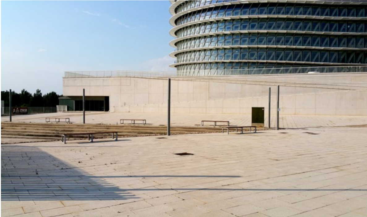
Figure 13. Torre del Agua actual condition view from Avenida Ranilla, ground floor entrance. July 2016 (photo D. Giordanelli, 2016).
