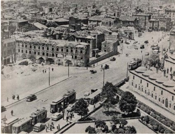
Figure 18. Istanbul. Simkeşhane and Ordu Avenue before the demolition (UNSAL 1968, p. 33).
